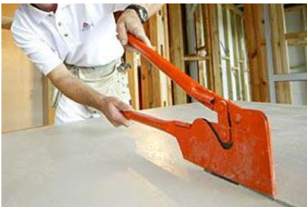
Cutting fibre cement sheets
