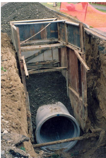
Trench excavation with steel shoring
