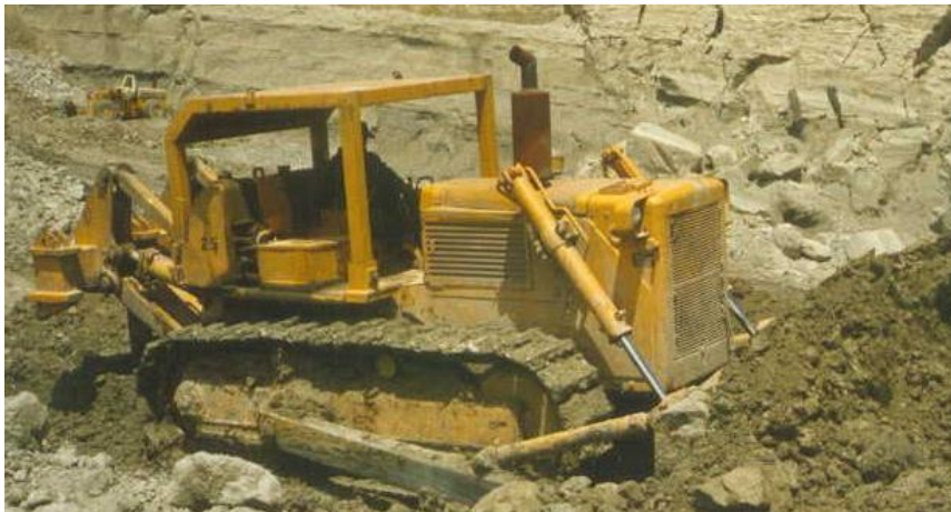
Bulldozers are used in site clearing and bulk earthworks
