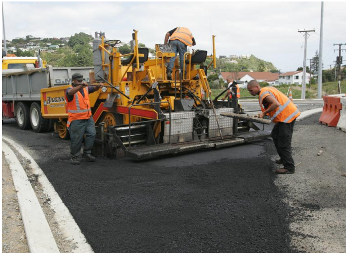
Surfacing with asphalt
