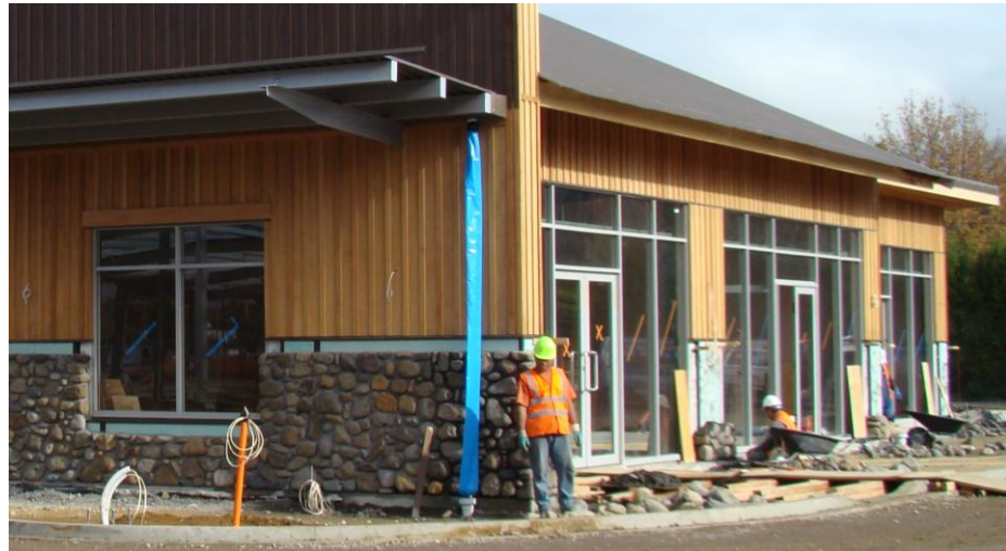
A joiner would have won the contract to make this joinery in the Bethlehem Town Centre
