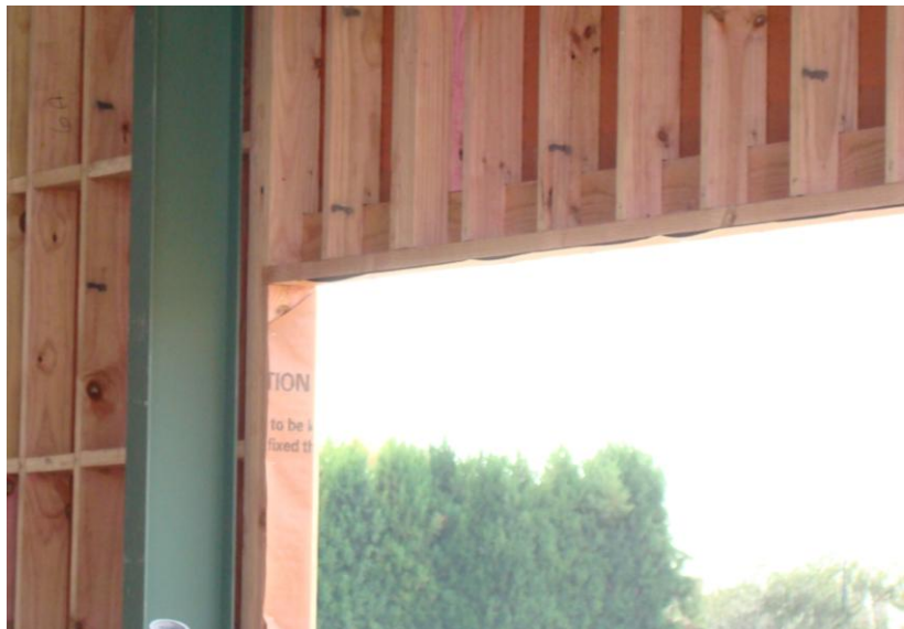
The framing and building paper is ready for the external cladding. Then the glass joinery is installed.
