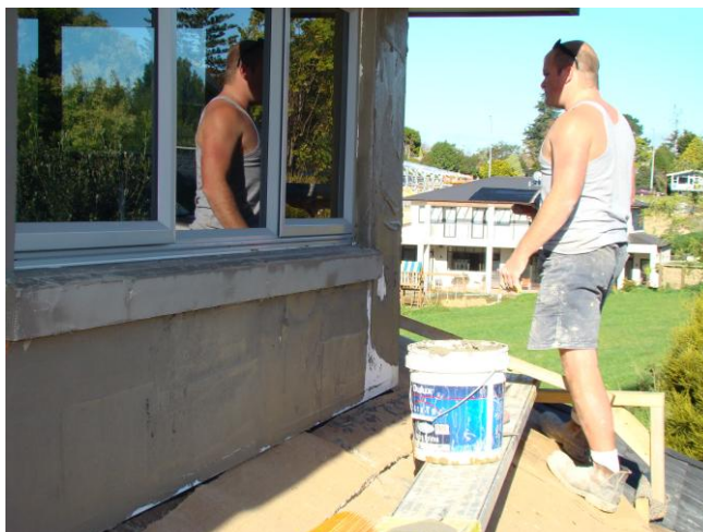
The plasterer finishes off the external cladding once the joinery is installed.
