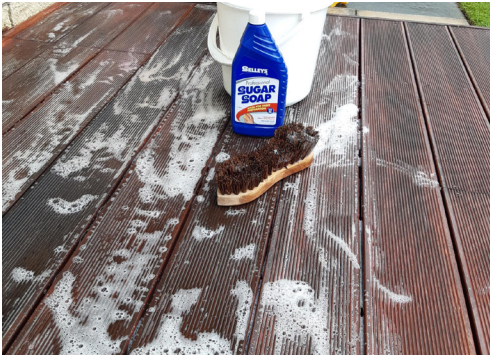
Washing a deck
