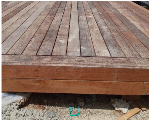
Provide adequate run-off for low decks
