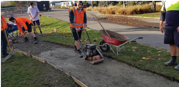
Compacting the bedding sand (left) and the finished paths (right).
