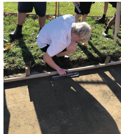
Flattening off and tidying up the crusher dust at the sides with the steel trowel
