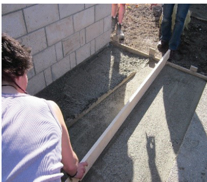
The screed board in progress. (left)
