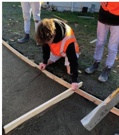
Flattening off and tidying up the crusher dust at the sides with the steel trowel
