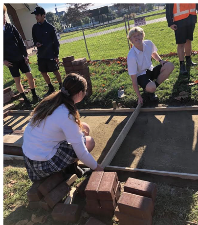
Note the gap between the inside boxing and the edge of the paver. A 20mm spacer was used with the first row.
