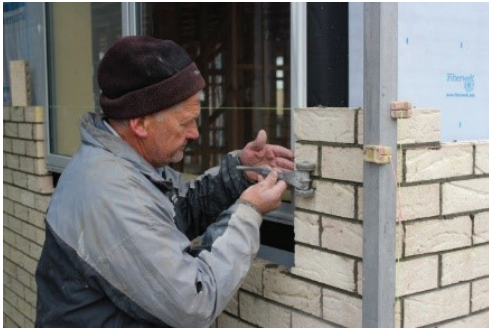
A wheeled raker being used.
