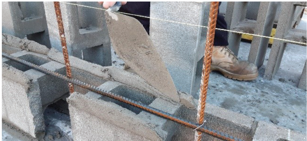
A trowel is being used to place the mortar ready to place the next course (line of bricks).
