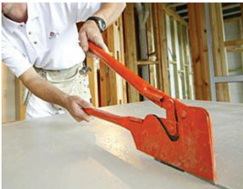
Cutting fibre cement sheets
